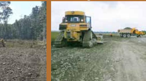
**Compacting levee embankment**
