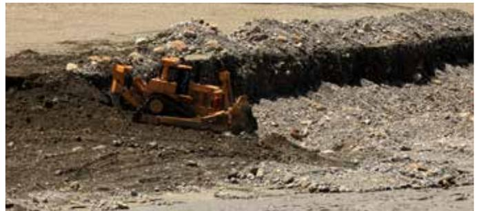
Levee construction sequence: PT-FI employs more than 75 haul trucks and 60 pieces of heavy equipment to support construction and maintenance of the levees to laterally contain the tailings within the deposition area footprint.
