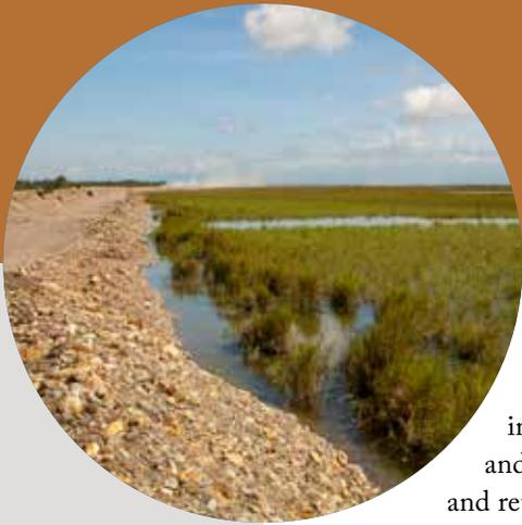
The buttress of the west levee, with *Phragmites karka* grass naturally established on deposited tailings sediments
