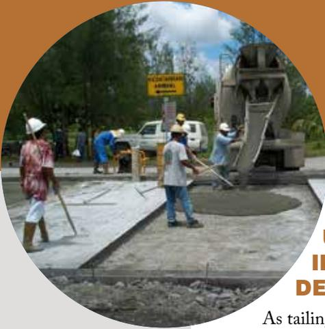
*Tailings concrete has been used for road construction in the Mimika Regency.*
