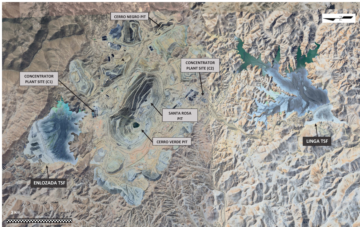
Figure 3. Cerro Verde Mine Site (March 2024).
