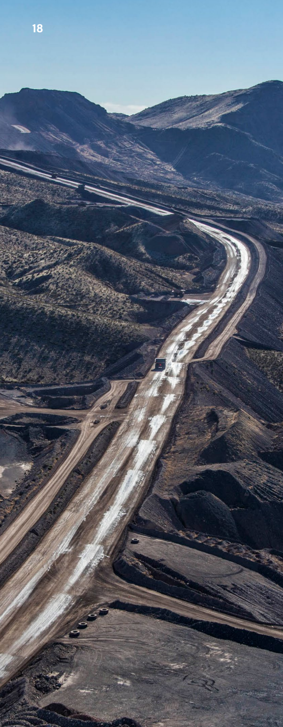
Safford is a mine-for-leach operation in Arizona that produces copper cathode. The operation consists of three open pits, including the Lone Star open-pit.
