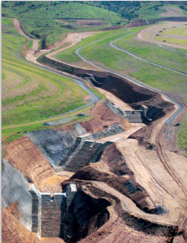
The Redrock Diversion drop structures were constructed as part of the award-winning reclamation project at Tyrone in New Mexico. These structures manage storm water from a large watershed between two reclaimed tailings dams.
