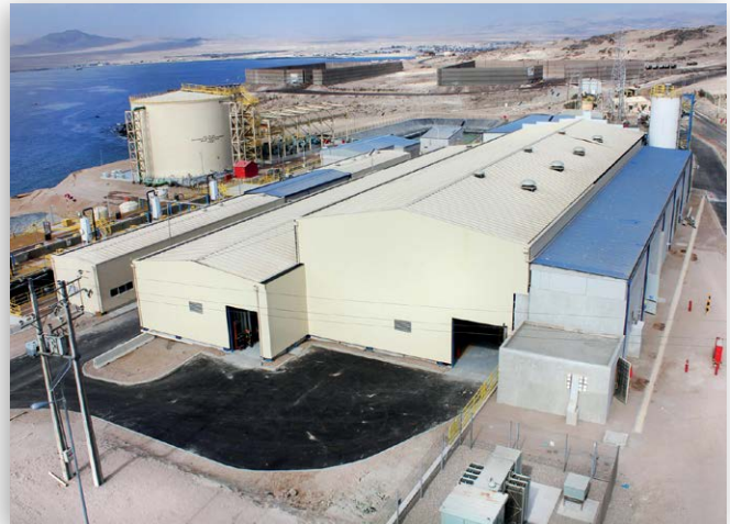
A desalination plant and pipeline will supply Candelaria’s longer-term water needs and has afforded the opportunity to transfer potable quality water rights to the local water utility for residential uses.
