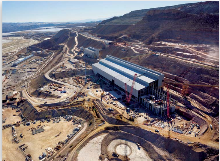
At our Morenci mine in Arizona, we are expanding mining and milling capacity to process additional sulfide ores. The new mill will use considerably less energy per ton of ore processed than older technologies.
