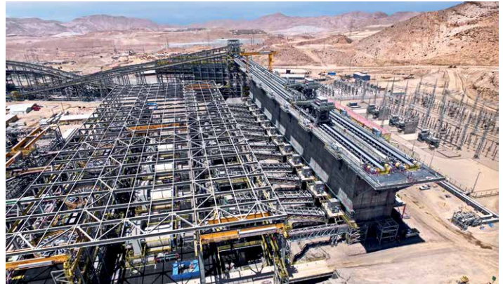
The Cerro Verde concentrator expansion includes a High Pressure Grinding Roll circuit that is approximately 40 percent more energy efficient than a traditional Semi-Autogenous Grinding mill circuit. The project tripled the concentrator facilities from 120,000 metric tons of ore per day to 360,000 metric tons of ore per day.
