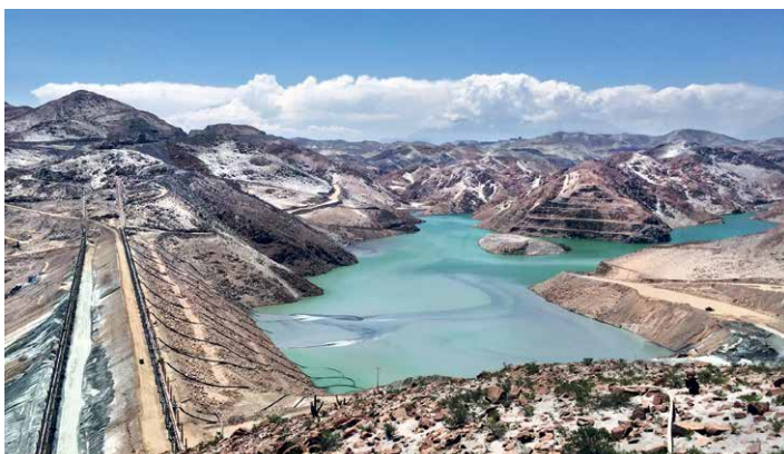
The new Linga TSF (above) and existing Enlozada TSF at Cerro are two of the largest TSFs in the global mining sector. Both were designed and built to withstand up to a 9.0 magnitude earthquake and withstand a Probable Maximum Flood.
