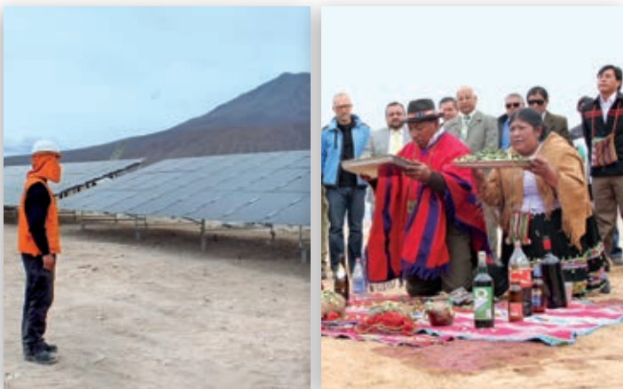
In 2014, El Abra partnered with a renewable energy developer to install 1,500 photovoltaic panels (left) and a wind turbine in the indigenous community of Ollagüe, Chile. Prior to the project the community relied solely on electricity from diesel generators. A traditional Quechua "Payment to the Earth" ceremony (right) is performed to give thanks for the project.
