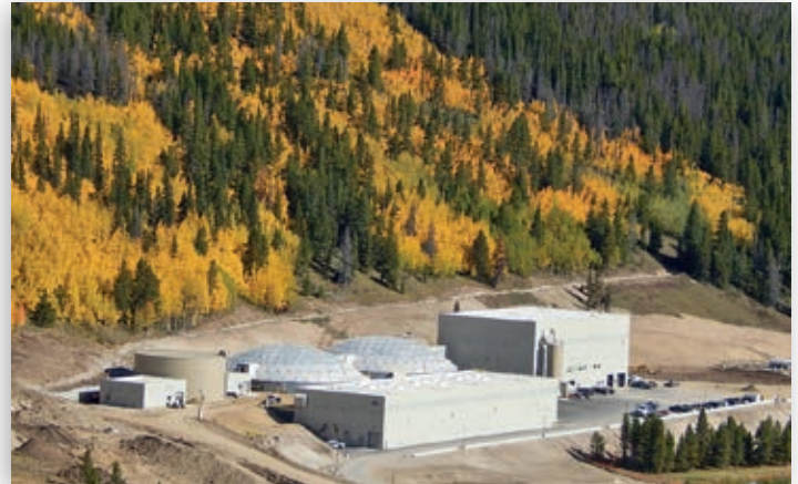
In July 2014, Climax Molybdenum’s state-of-the-art water treatment facility began operations to treat up to 14,000 gallons per minute from the Mayflower Tailings Storage Facility. The treated water is discharged into Ten Mile Creek, which supports local fisheries and recreation areas in Summit County, Colorado.
