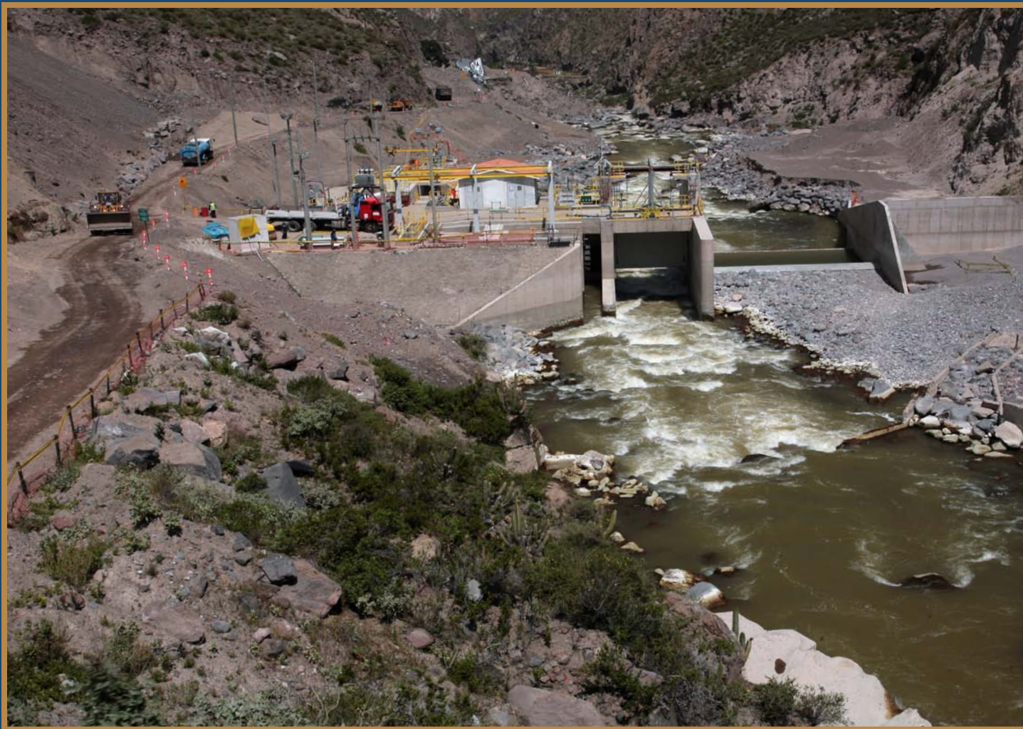
Plant intake structure for new potable water treatment plant
