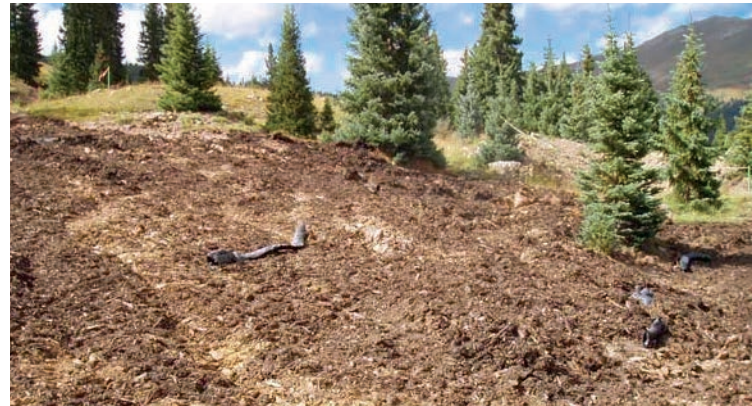
Same site after placement of soil cover, seed and mulch.
