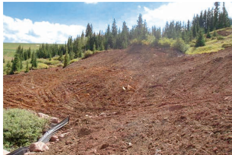
Reclaimed Lower Michigan mine following removal of acid generating waste rock.
