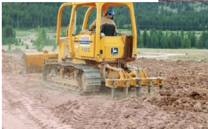
Reclamation of the Robinson Tailings Pond in Colorado. Clockwise from top left: tailings are capped with waste rock or overburden from our Climax molybdenum mine; a blend of biosolids and lime are blended into the cap material; surface is ripped and prepared for seeding to encourage vegetation growth.
