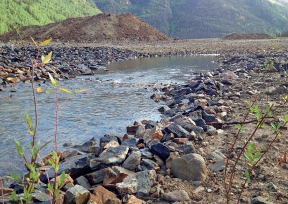
Reconstructed Woods Creek channel across lower URAD tailings impoundment.
