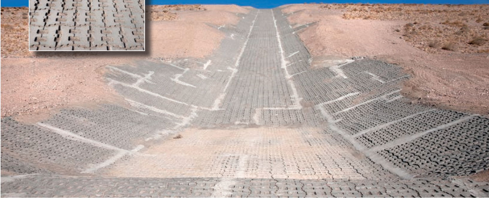
Articulated concrete block rises up Chino's tailings dam 700 feet to help prevent erosion in managing stormwater runoff. Photo inset: Close-up of concrete block.
