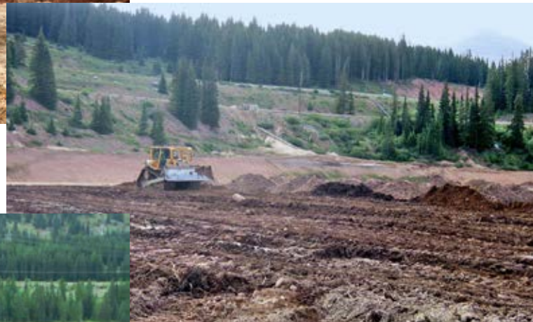
Reclamation of the Robinson Tailings Pond in Colorado. Clockwise from top left: tailings are capped with waste rock or overburden from our Climax molybdenum mine; a blend of biosolids and lime are blended into the cap material; surface is ripped and prepared for seeding to encourage vegetation growth.
