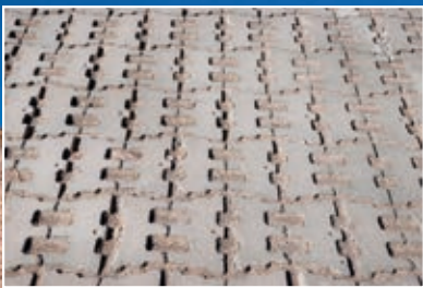
Articulated concrete block rises up Chino's tailings dam 700 feet to help prevent erosion in managing stormwater runoff. Photo inset: Close-up of concrete block.
