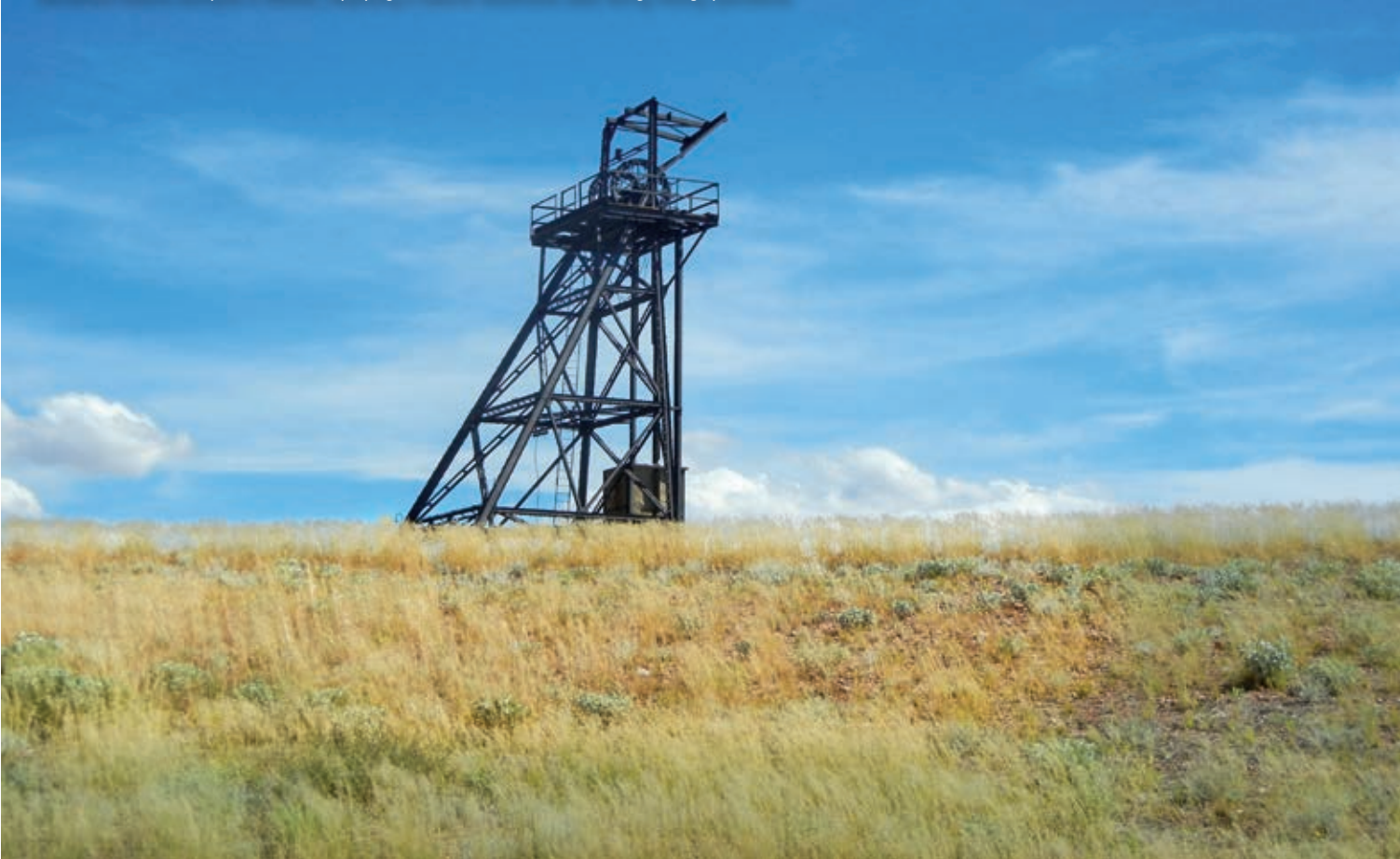
Reclaimed Galena stockpile in Bisbee, displaying a historic headframe used during mining operations.
