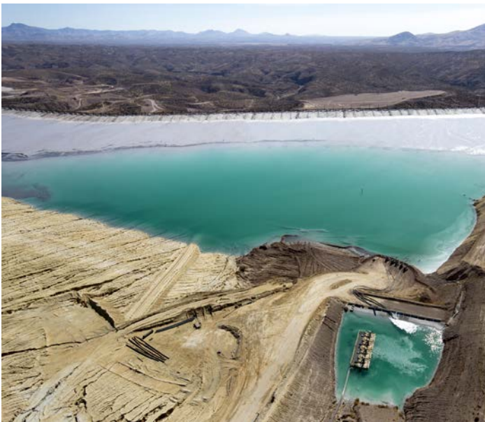
The majority of our recycled water originates from reclaimed water captured at tailings facilities and leach pads. Above, water on the Morenci tailing impoundment is set to be recycled.
