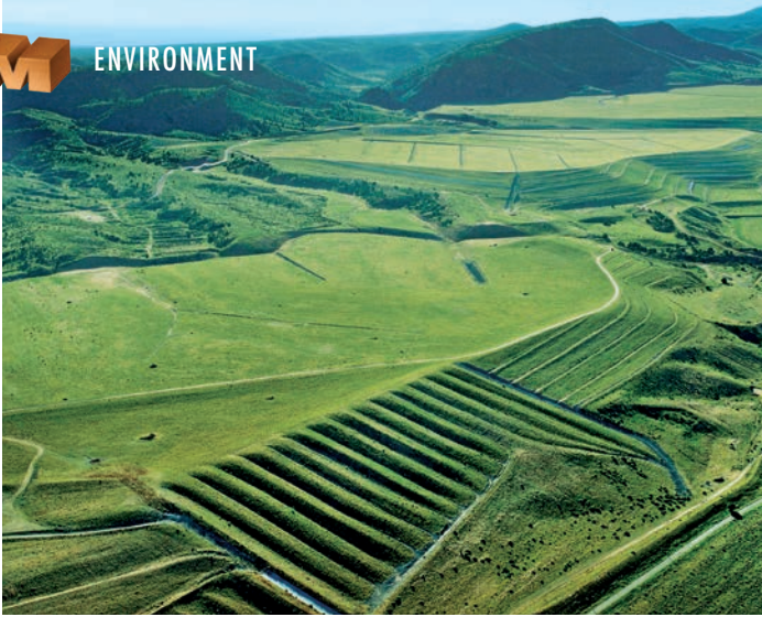
We reclaim inactive TSFs by regrading slopes, conveying and diverting storm water, capping with soil cover, and reseeding with native grasses and shrubs. Above are Tyrone TSFs in New Mexico after completing reclamation.
