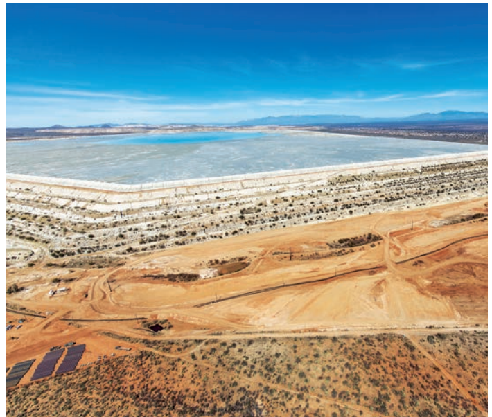
Active TSFs are continually monitored for embankment dam structural stability and environmental aspects such as dust generation potential. Above, buttress construction provides additional stability at the Sierrita TSF near Green Valley, Arizona.
