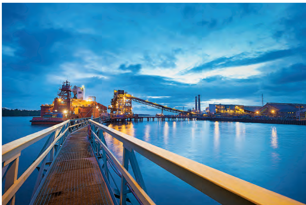
Copper concentrate is loaded at Port Amamapare at our Grasberg mining operation in Papua, Indonesia. PTFI is one of the largest taxpayers in Indonesia and has contributed over $60 billion to the country's GDP since 1992.
