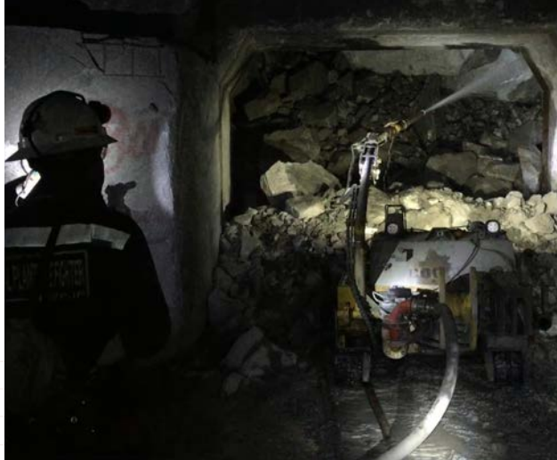
PTFI is developing and utilizing improved critical controls including water cannons to effectively move large boulders that may obstruct ore draw points while the operator maintains a safe distance.
