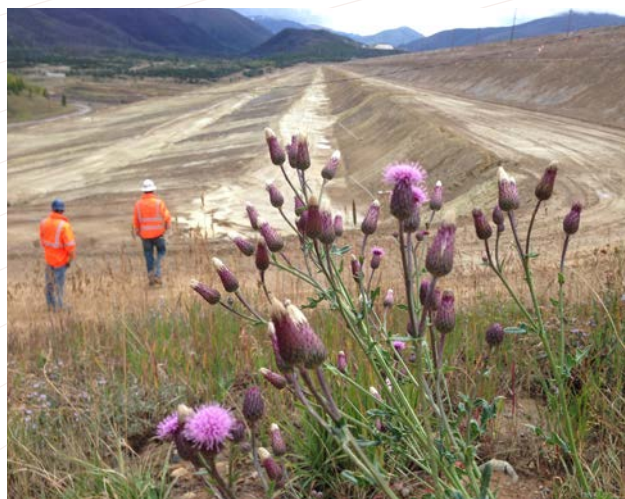
Members of the TST inspect the Henderson Tailings Dam in Colorado.
