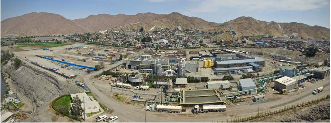
Utilizing its formal grievance system, Cerro Verde has successfully worked with community members, including within the Uchumayo District (photo background), to address 146 complaints regarding noise and vibrations from pumping stations (photo center). The stations are an integral component of the Arequipa Region's first ever wastewater treatment system which is designed to treat 90 percent of Arequipa's domestic and industrial wastewater. Grievance remedies ranged from home relocations to replacement of windows.
