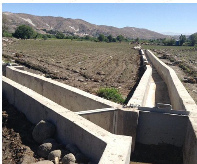
Cerro Verde continues to provide financial and technical support for water-efficient crop irrigation systems in nearby communities. More than 440 local farming families are now utilizing over 27 kilometers of lined irrigation channels to prevent excess water loss.
