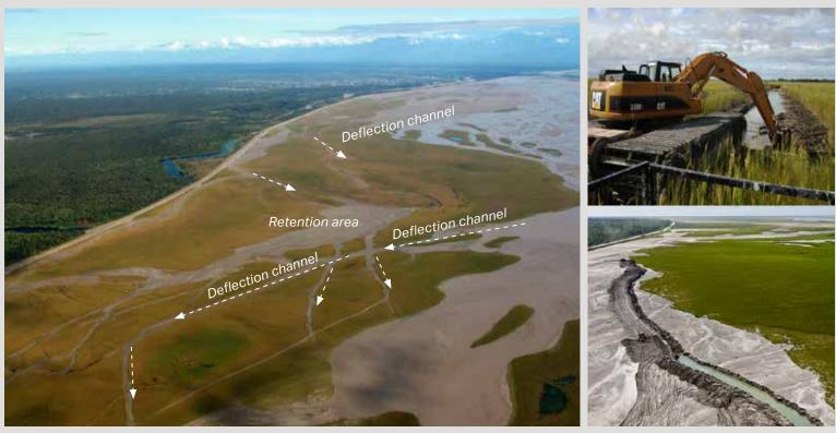
PT-FI's fill back swamp program involves the use of a swamp excavator (*top right*) to create channels (*bottom right*) that deflect tailings flow into lower elevation zones within the tailings deposition area, slowing stream velocity and increasing tailings retention (*left*).
