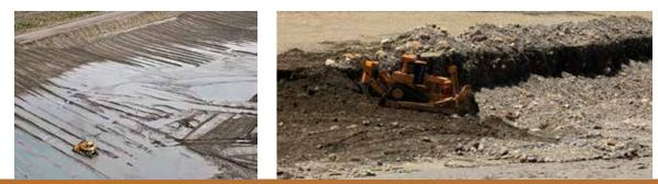
Levee construction sequence: PT-FI employs more than 75 haul trucks and 60 pieces of heavy equipment to support construction and maintenance of the levees to laterally contain the tailings within the deposition area footprint.
